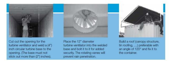
The container should be retrofitted, as in the below diagram. The pointed roof (at a 120-degree angle) is preferable, as it will provide better protection from heavy rain.
