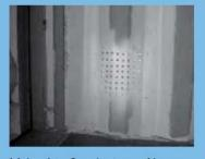
Make 4 to 8 rodent proof lower lateral 12" x 12" air vents by drilling series of ½" holes through the inner groove of the container wall. (Inside view)
