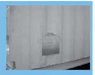
Cover these air vents on the outside with home made moulded galvanized steel plates welded ¾ around to prevent vertical & lateral water infiltration.
