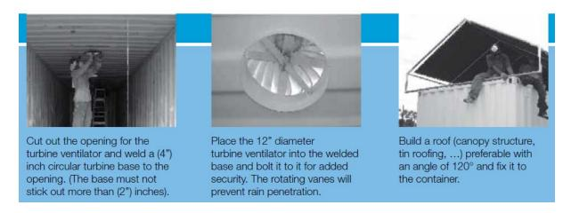
The container should be retrofitted, as in the below diagram. The pointed roof (at a 120-degree angle) is preferable, as it will provide better protection from heavy rain.
