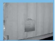
Cover these air vents on the outside with home made moulded galvanized steel plates welded ¾ around to prevent vertical & lateral water infiltration.
