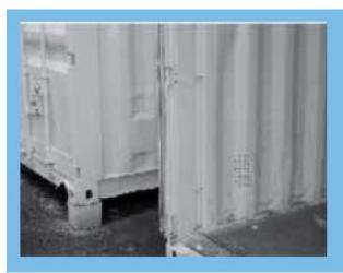
Apply 2 coats of anti-corrosion white paint inside and outside the container. Cover the air vents on the inside with mosquito screening to prevent insect infestation.
